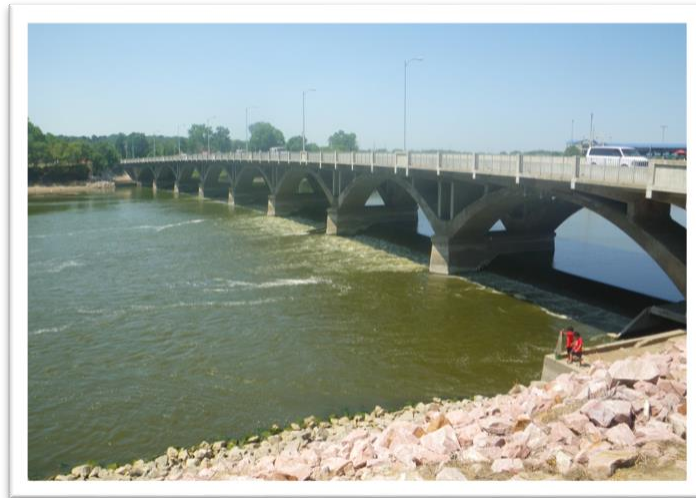
The Center Street Dam in its current state.
